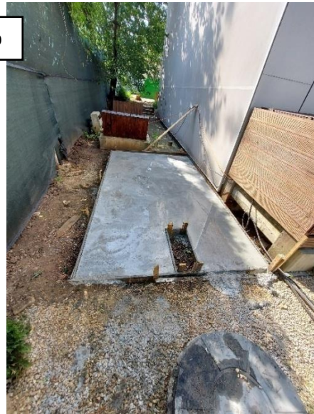
Figure 7. Concrete foundation for the container (a – before, and b – after)
