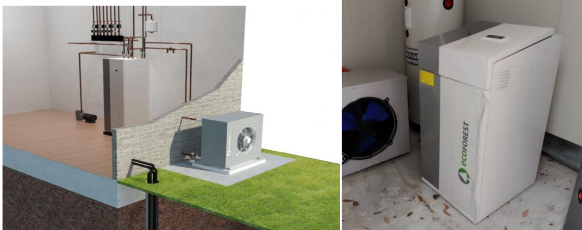
Figure 1. Heat pump equipment used for the proposed system
